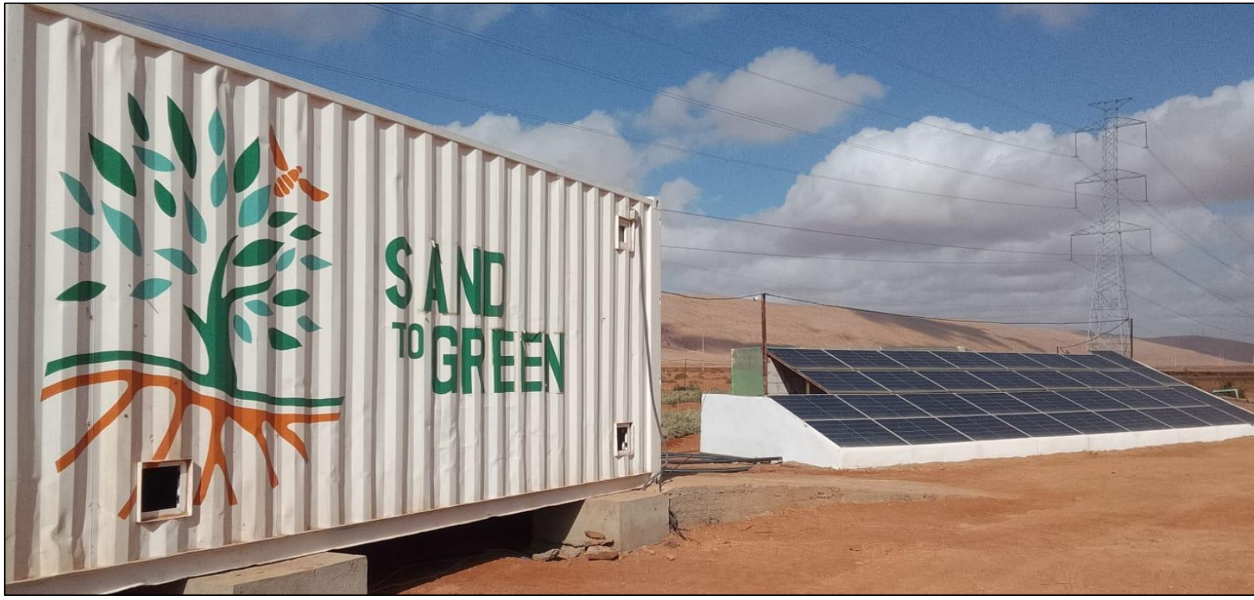
Fig. 2. Solar-powered Mascara Osmosun desalination unit, producing 6 m³/h
